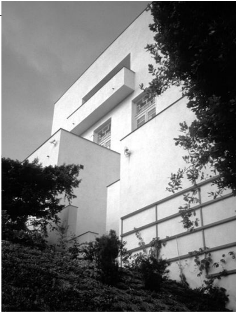
Adolf Loos, Müller Villa, Prague, 1928–29. Rear of the house seen from below. Photograph by the author.
