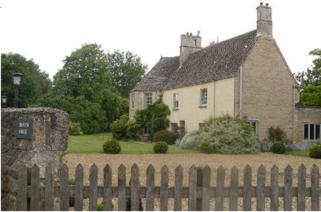
Another view of the house
