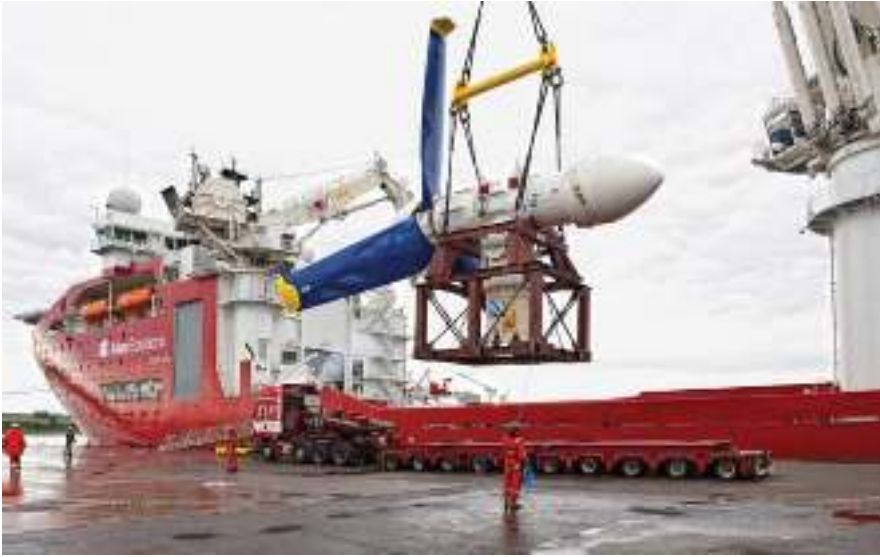
Figure 1.2 Transporting a tidal stream turbine (Atlantis Resources; Mike Roper (photographer)).
