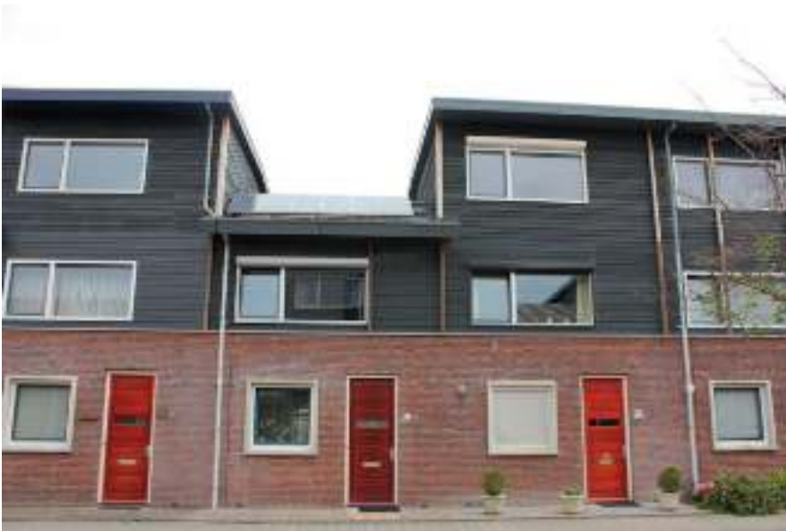
Fig. 1.8 Solar powered homes in Alkmaar, the Netherlands
