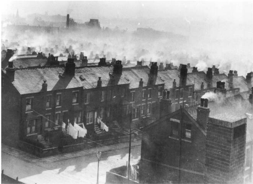
▲ 0.2 Back-to-back housing in Leeds
