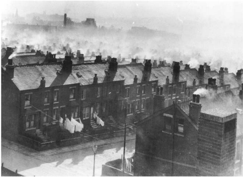
▲ 0.2 Back-to-back housing in Leeds
