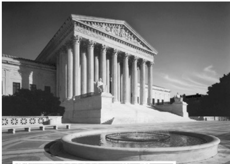
The west façade of the Supreme Court building, c. 1992.
